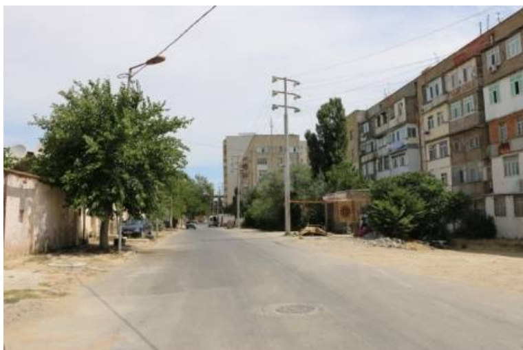
4- 5 - storey buildings built in the past (during Soviet times)
