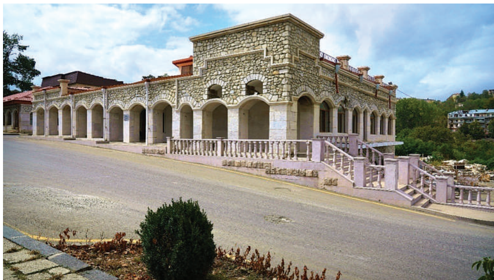
Fig. 2. Caravanserai of Agha Gahraman Mirsiyab.
