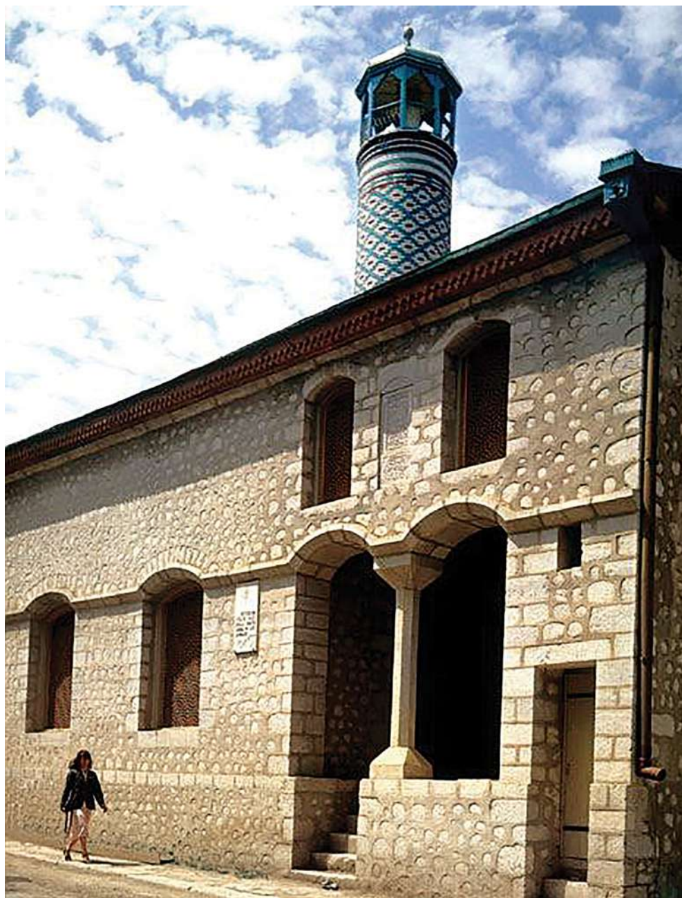
Fig. 3. Restoration of Saatli mosque.
